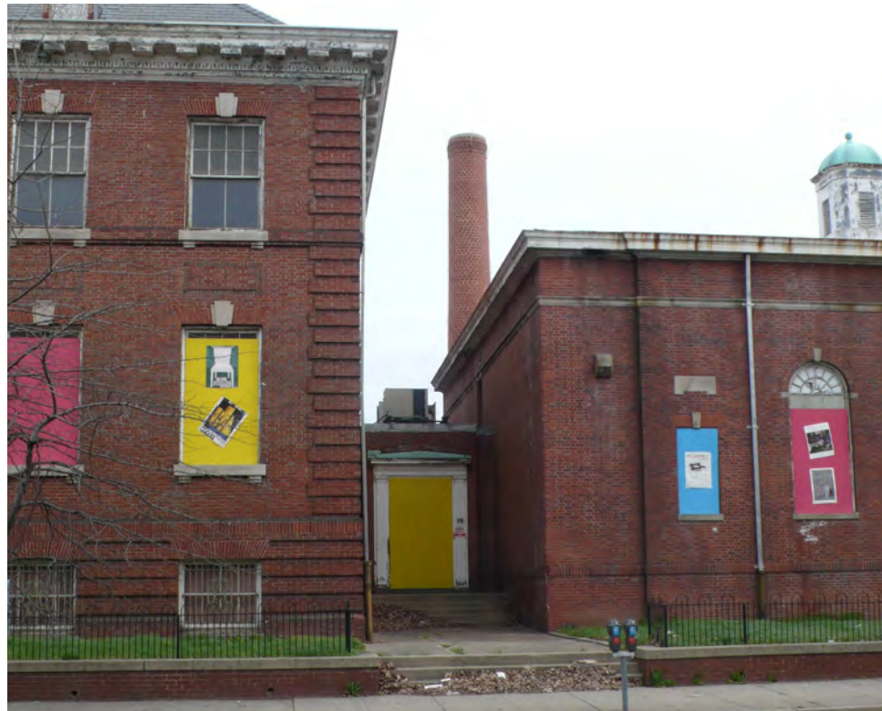
2 Randall School I Street facade between main building and auditorium
